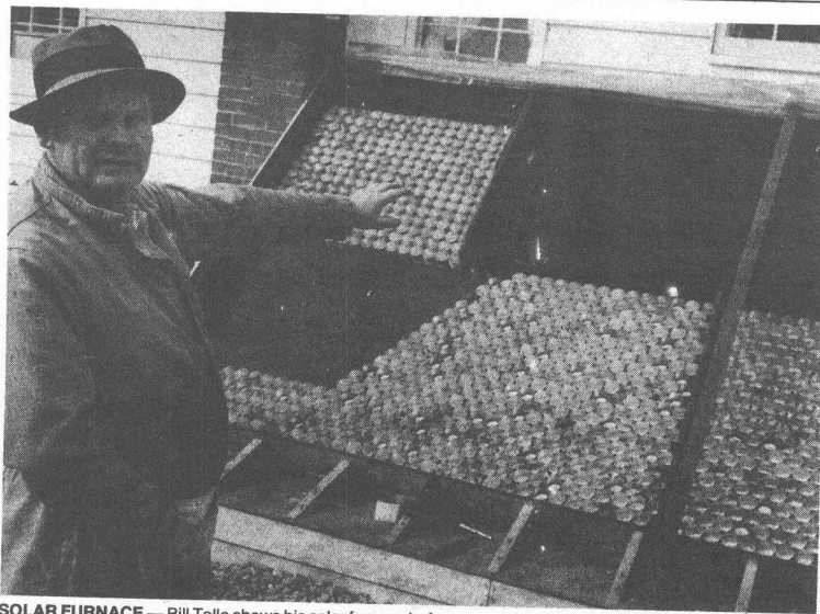
SOLAR FURNACE — Bill Tolle shows his solar furnace before completion. The black cans absorb heat from the sun and warm the air between the cans. The air is then circulated into the basement and the rest of the home via ducts. [Photo courtesy the Middletown, Ohio, Journal of Feb. 9]
